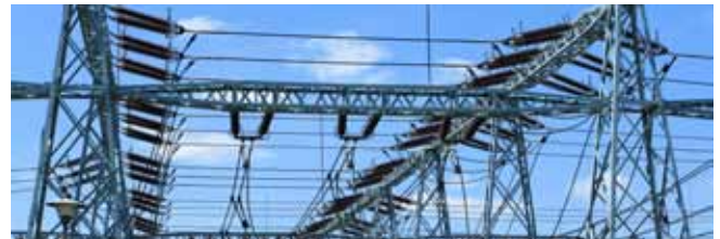
Modernisation and extension of electricity networks of ENEA Operator.
